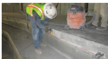
After: Concrete grinding.
